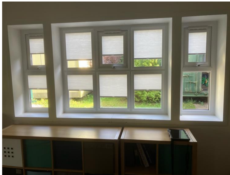
Image 14: New windows at Bedminster Quakers Meeting House
