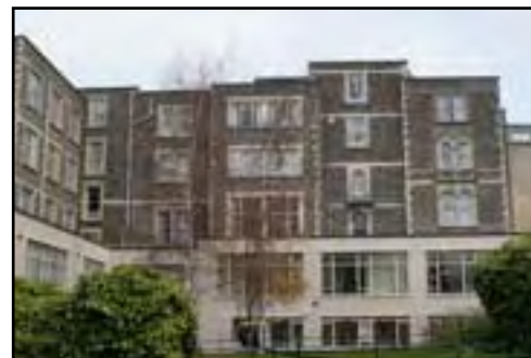
South elevation has lost rhythm through changed window openings from vertical to horizontal emphasis
