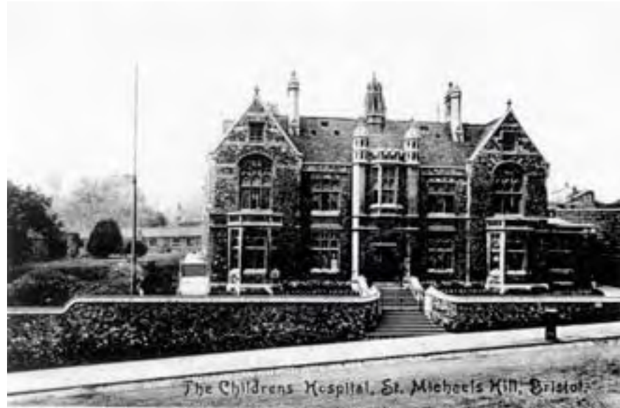
The front elevation of the building shown in an early postcard. Whilst the elevation survives fairly well intact, the cupola over the main entrance has been lost.
