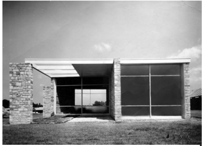
The Gane Pavilion by Marcel Breuer, Ashton Court
