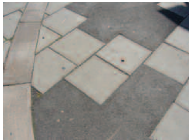
Figure 46: Mix of street surfaces, Colston Street
