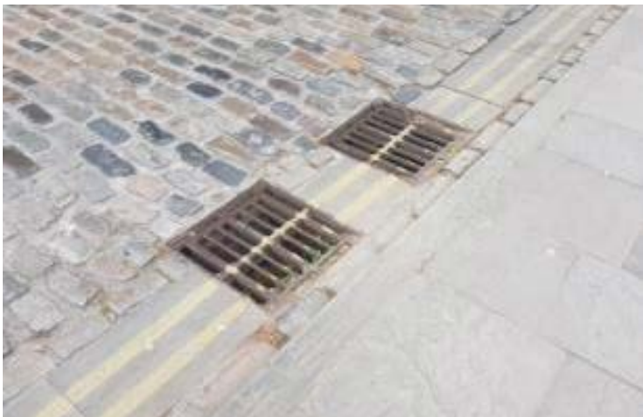
Fig 3: Heel guard gully cover in footway
