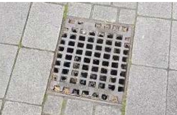
Fig 3: Heel guard gully cover in footway
