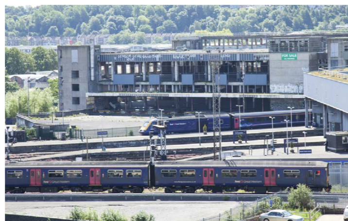
Poor first impression of the city, particularly the view of the Former Royal Mail Sorting Office
