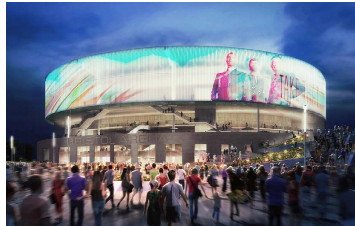
Bristol Arena will open in 2018 and will become one of the city and the region's most important places of assembly, setting a new benchmark for arena design
