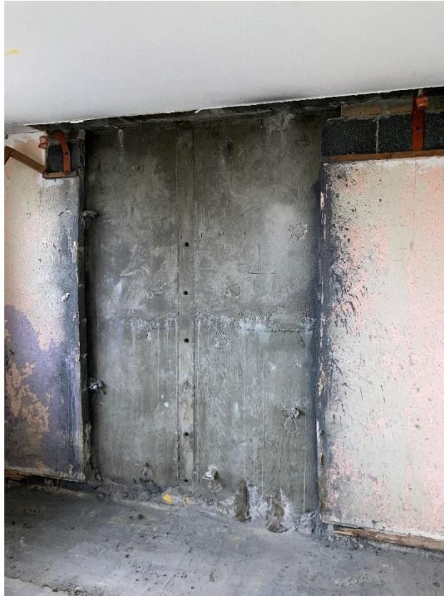
Photograph 7: External (Flank) Wall Cast In-situ Panel with Masonry Wall
