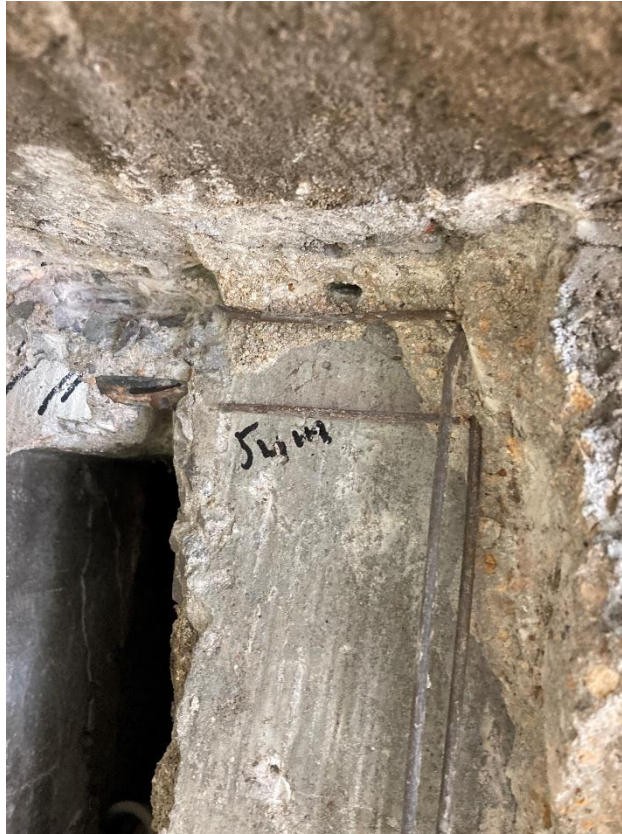
Photograph 5: Typical Layer of Shotcrete in front of Low Cover Panel
