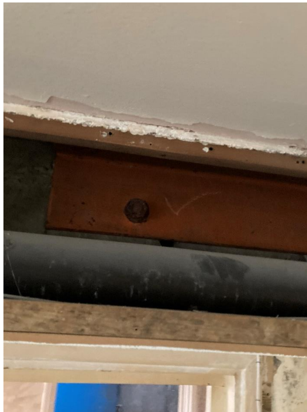
Photograph 4: Typical Temporary Support Angles
