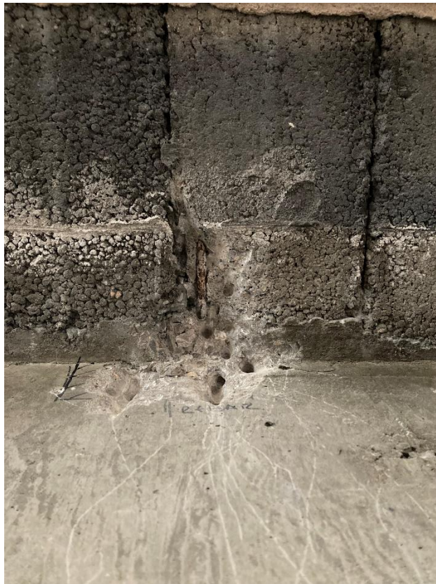
Photograph 8: Precast Floor Beams Reinforcement Provision
