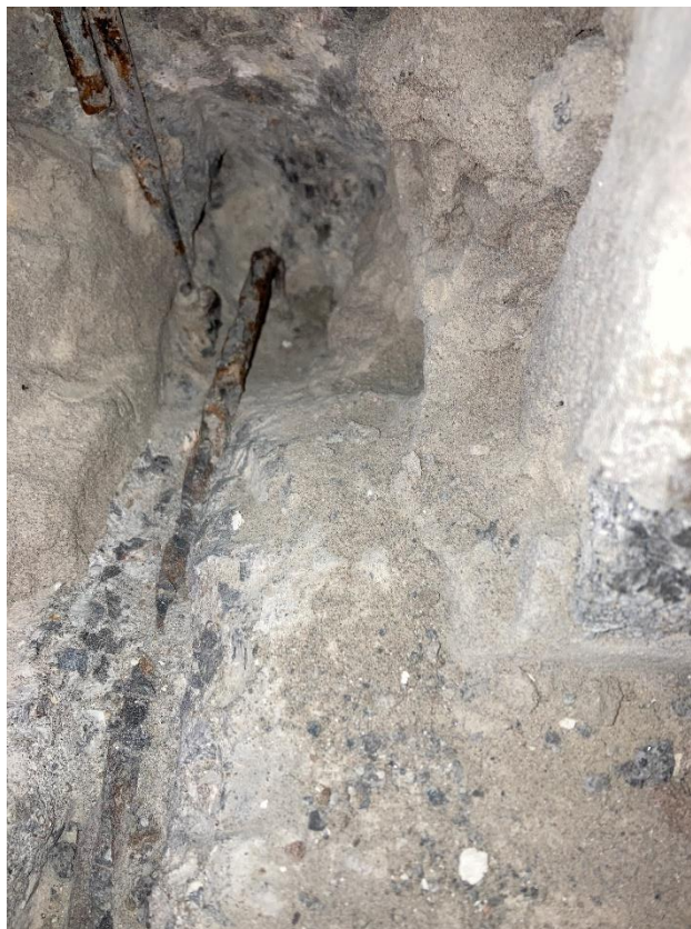
Photograph 2: External Wall Junction Horizontal Tie
