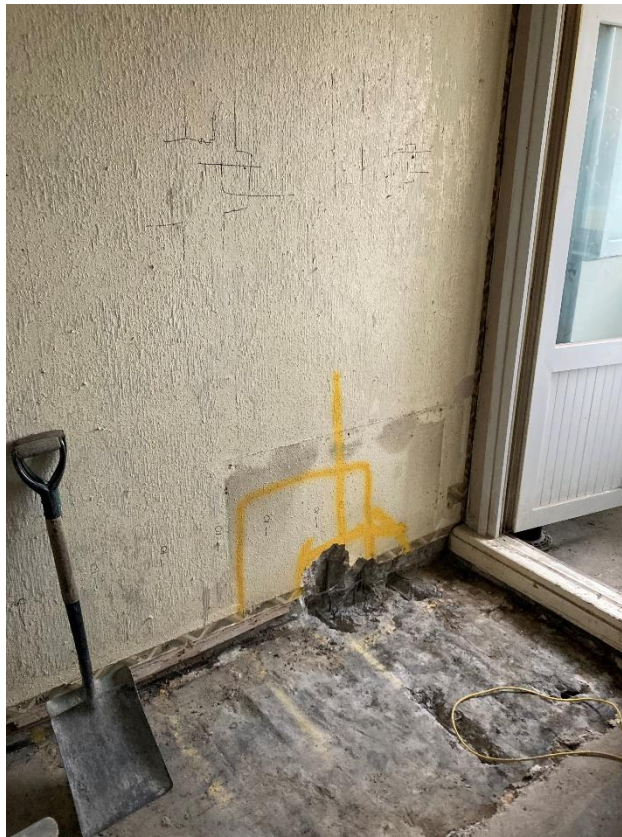
Photograph 1: Internal Wall Junction Horizontal Tie
