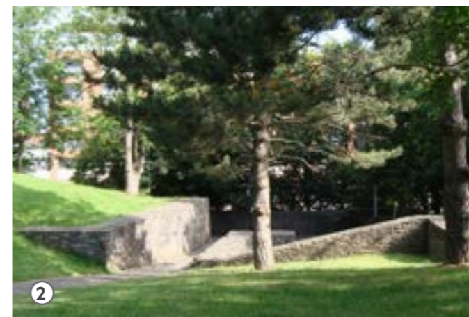
Fig. 94 Existing walls within Castle Park
