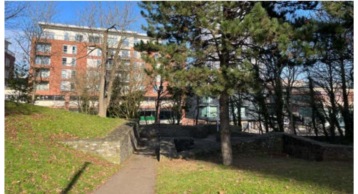
Fig.139 Site Photo - Entrance to Broad Weir
