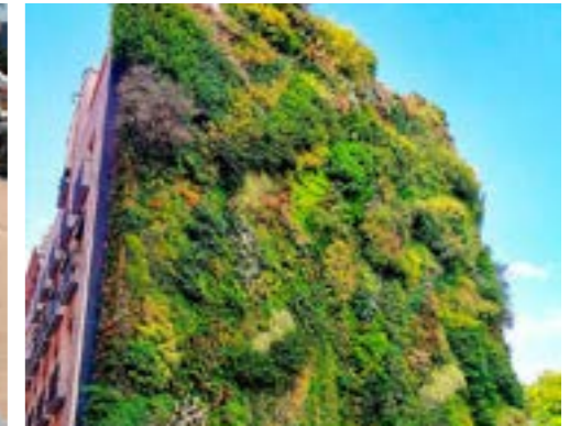
Frontage to Castle Park - Biodiverse Vertical Greening
