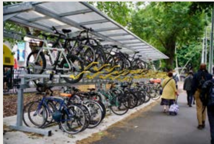
Figure 95 Two level cycle parking
