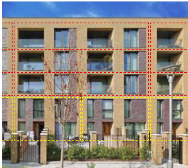
Figure 173 Modern residential block with front door maisonettes on the lower two floors and internally accessed apartments on the upper floors
