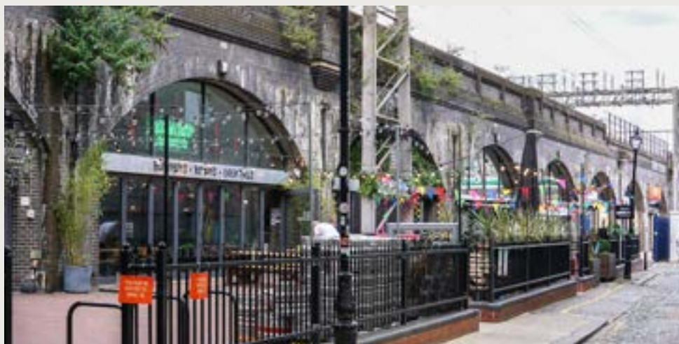
Figure 128 Activated heritage arches
