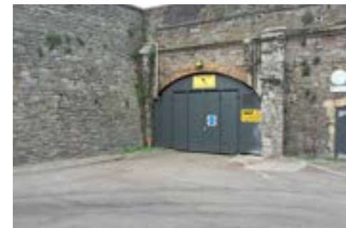
Figure 122 Bristol & Exeter Yard rail replacement area
