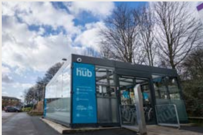
Figure 94 Containerised cycle parking
