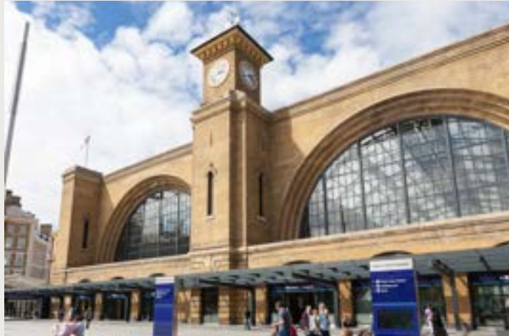
Figure 92 King's Cross station
