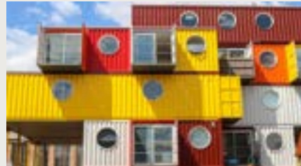
Shipping container offices
