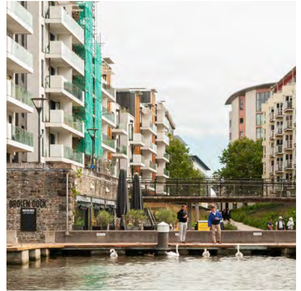
Photographs of St Augustine's Reach and Harbour Inlet (Source: DK-CM)
