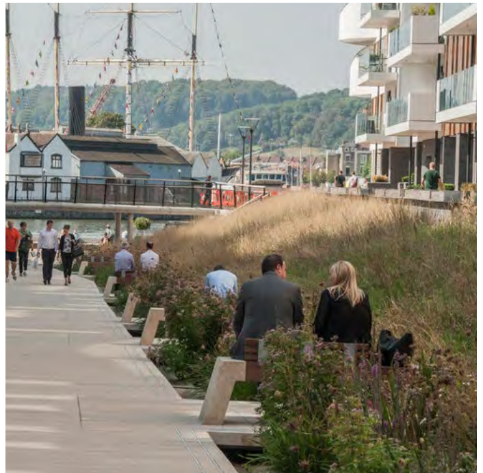
HRP1: Integration of SuDS and seating into walkway and public realm in Bristol. (Source: GA Photo_hyc)
