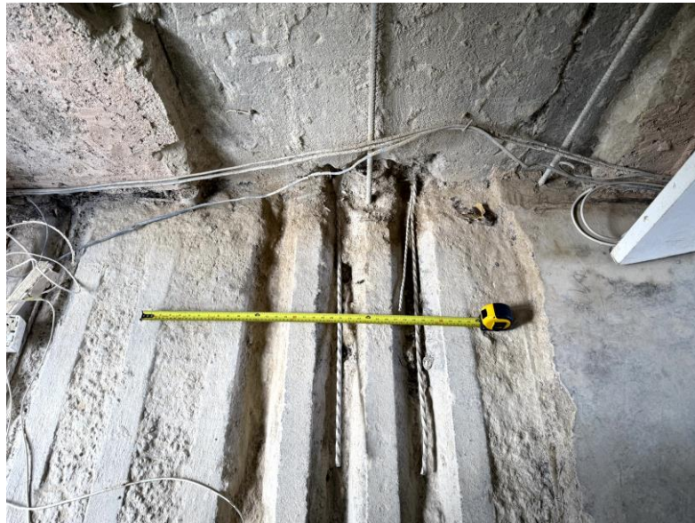
Figure 16 - Shotcrete lining with reinforcing projecting through the floor.
