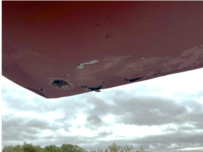
Figure 13 - Place Holder Images for balcony spalling reinforcement
