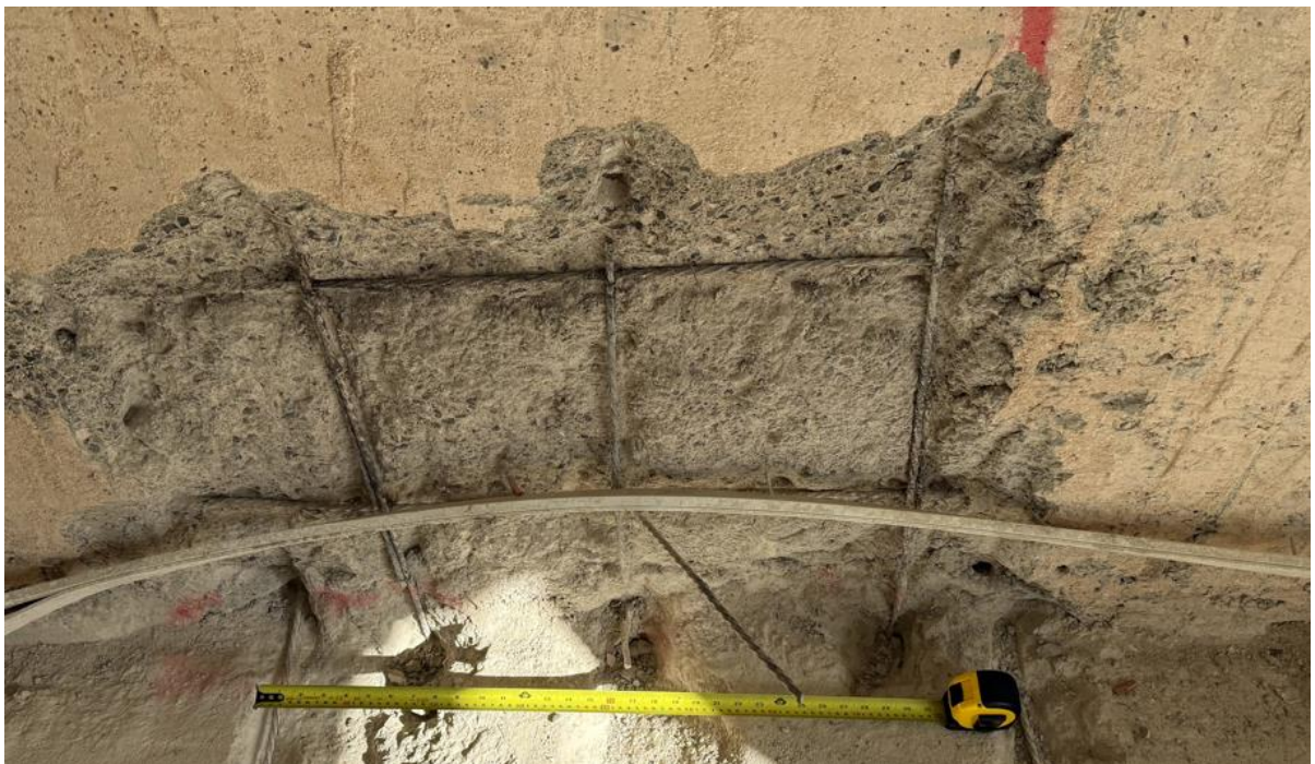
Figure 13 – Langton House intrusive wall investigations
