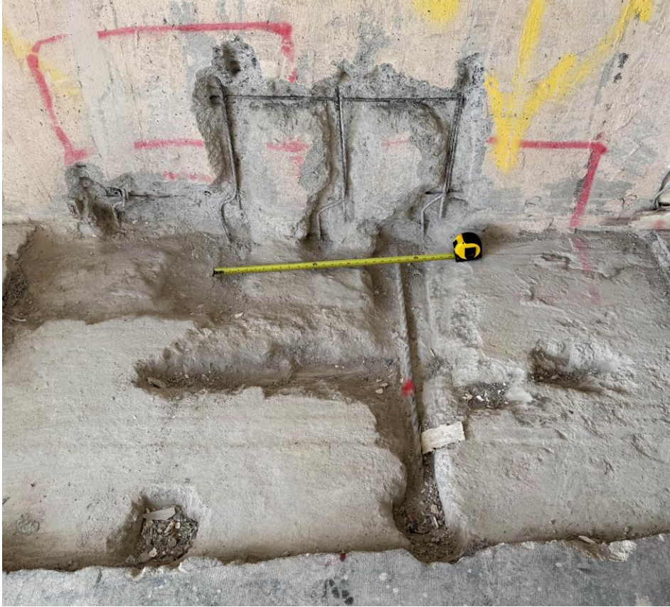
Figure 8 - Floor to wall opening up works in Langton House
